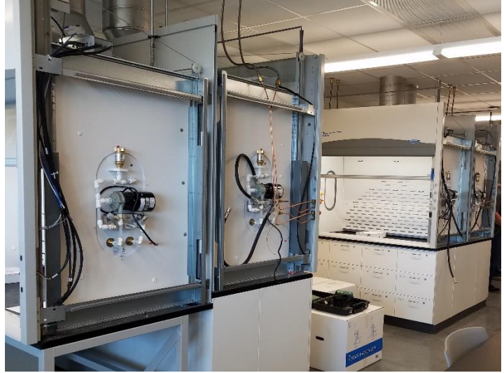
Back side of EcoDenser with hood panel removed
